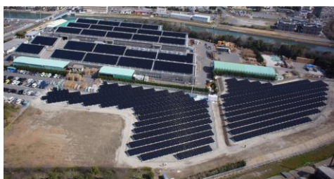
Fig. 1 1.3MWdc CdTe PV system at Kitakyushu-shi in Japan
